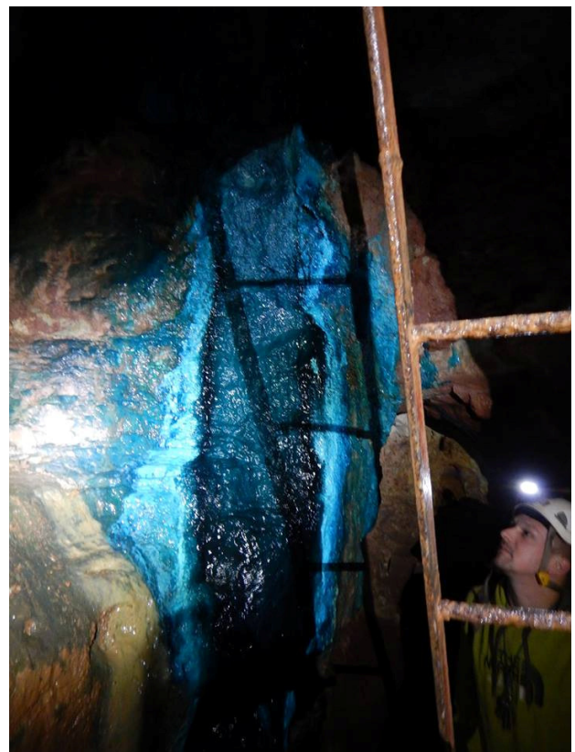
Copper deposit around the ladder sections (Ed for scale)
